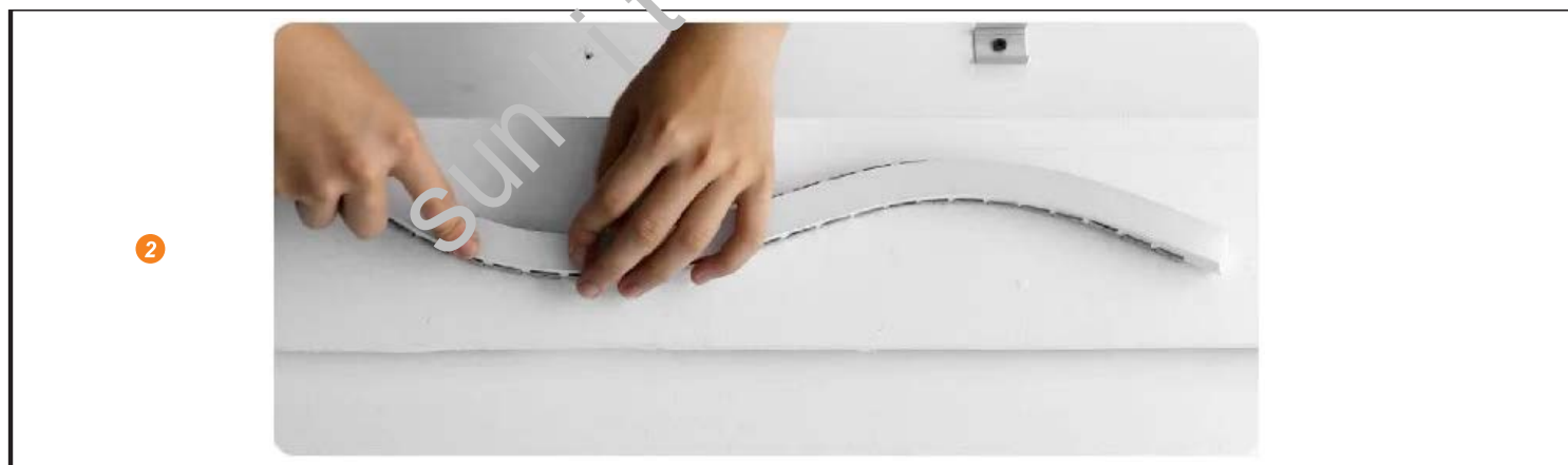
2 Fix the neon tube into the flexible keel according to the shape
