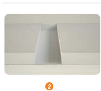
2 Grooving the location for installing neon tubes
