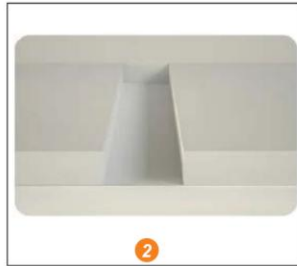
Grooving the location for installing neon tubes
