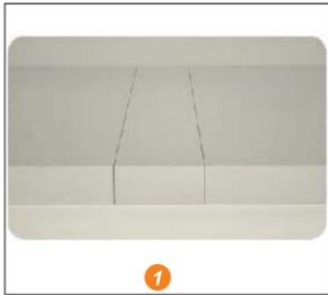
Measure the location of neon tubes to be installed
