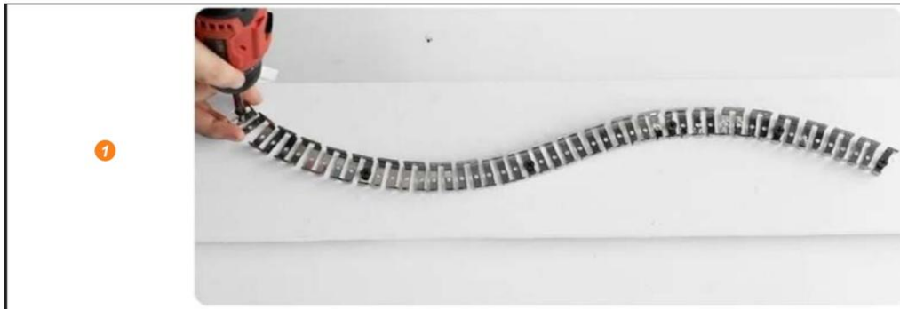
1 Use screws to fix the flexible keel according to customized styling requirements
